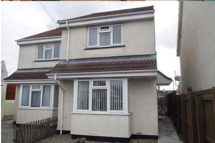
149 & 151 Barton Hill Road – 2 x two bed houses
