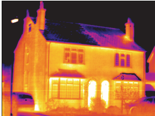
Figure 5: External thermal image of two semi-detached houses
